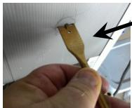
Now, using your hands or the hand-powered drill only, turn the spade bit slowly to slice through the insulation backing and make the hole. When you get through the backing, go slowly through the insulation, just in case you missed detecting a refrigerant line.
