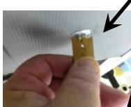
Coming in from the outside, ream out the insulating material. Stop just as you hit the interior liner. Twist a few turns to scribe the plastic liner, then look inside and inspect from there. Insert the spade bit from inside the refrigerator, give it a couple of twists to scribe the hole's edges, then withdraw and finish the hole from the back. De-burr both holes with a pocket knife and insert both grommets. Hopefully you'll have a nice, clean, professional-looking installation.
