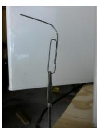
Straighten one leg of a paper clip 90 degrees. Stick it into the hole that you just drilled. Push it in until either you feel resistance from a refrigerant line (*Whew! You located it without drilling it!*) or until you hit the inside wall. Now, rotate the paper clip, probing in and out, making sure that there is no refrigerant line nearby. We’ll be drilling a 1” or less. If you find a line, just offset your next small hole so as to miss it, then repeat until you find a clear area.
